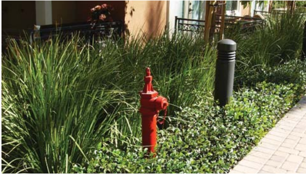
Figure 2-26: Standpipe
